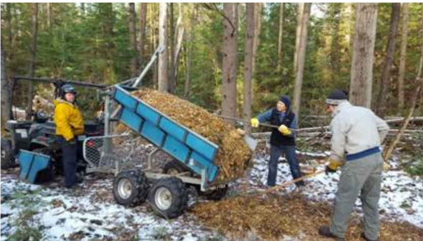
Spreading wood chips on the new R loop "re-route" trail
