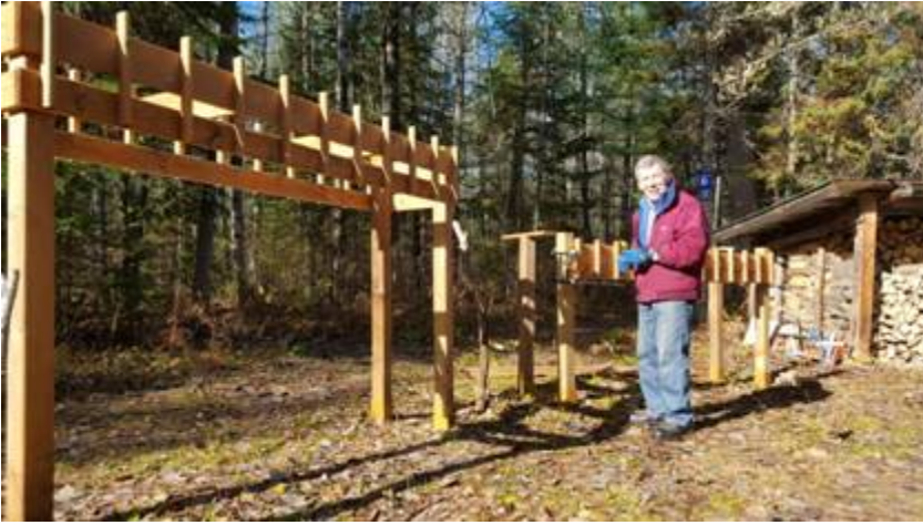
Designing and building new ski racks next to the chalet
