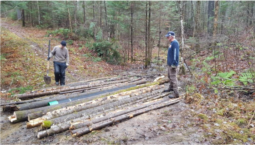
New culvert at the base of the big M hill
