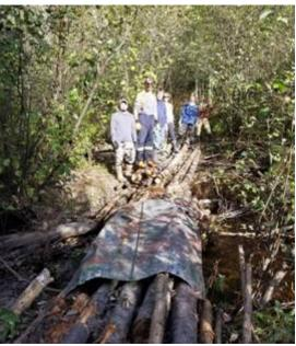
P loop crossing: It takes a big crew to move those big logs! This crossing on P loop needed rework after the spring runoff carried away some bits. Deadfalls scavenged from the bush make convenient construction materials.
