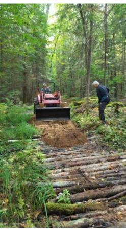
R loop drainage: Sections of R loop near the river are perpetually wet with marsh runoff (left photo). A revolving crew of volunteers have cut ditches, laid drainage pipes, cut and laid logs for corduroy, and covered it all with sand (right photo). That should take care of the largest ice patches that skiers have struggled with in the past.
