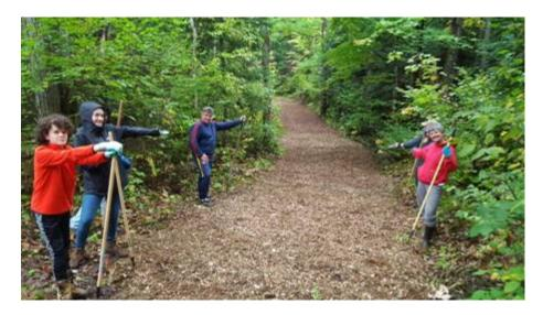
M loop resurfacing: Welcome to M loop! Local tree services and utilities deposit free wood chips behind the chalet. Volunteers have brought the chips out to Short M with tractor-loader, trucks, ATV, and dumping trailers, and have raked it all smooth. Skate-skiers will find Short M less lumpy this winter.
