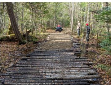
Example of trail improvements in 2022 Oct-Nov. Left: original wet area on R Loop. Right: corduroy (cut from excess balsam) placed over area and then smoothed over with gravel.
