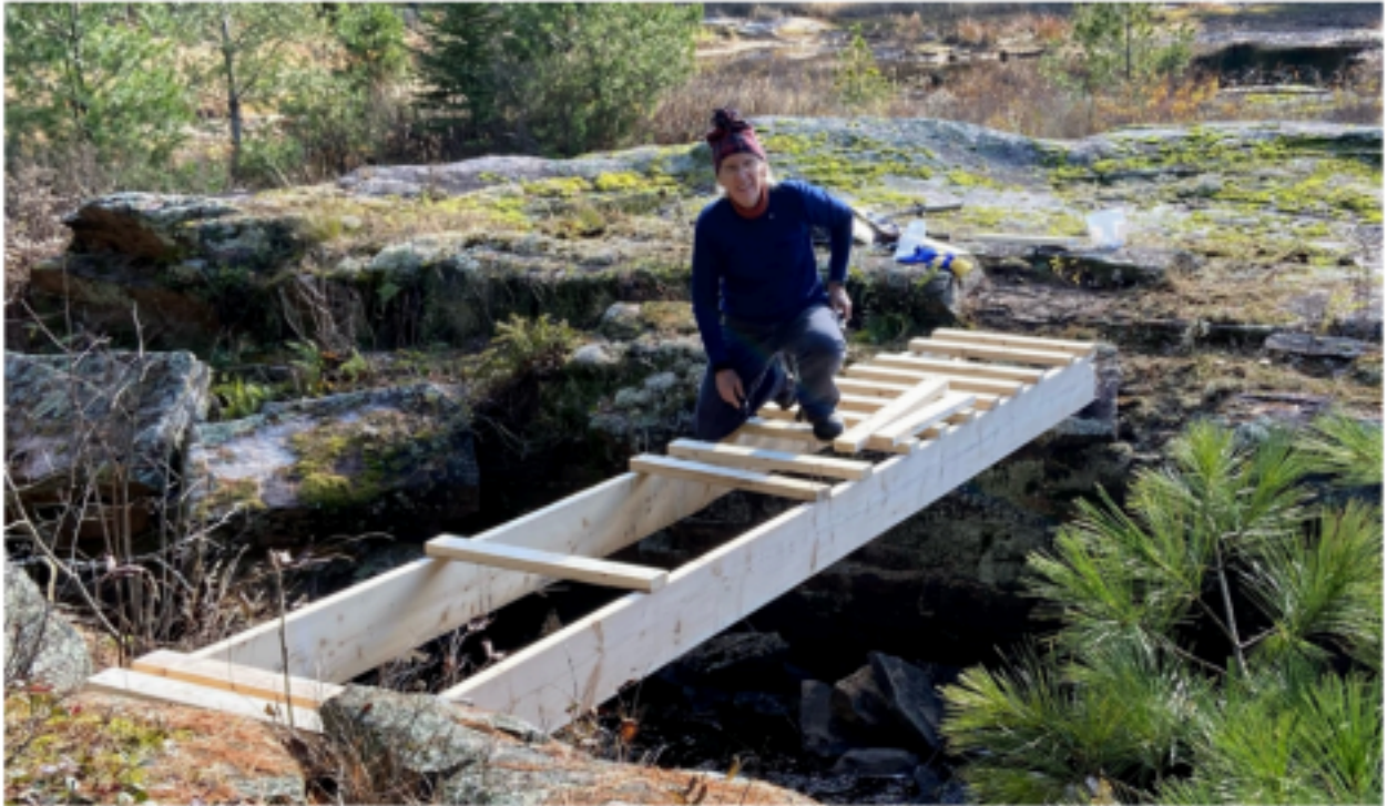
Karen Collins working on the New Bridge near the Cabin
