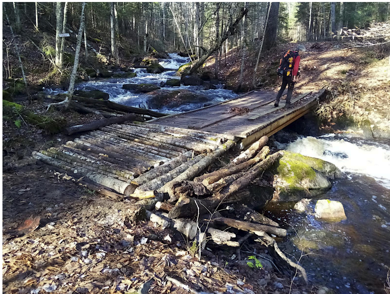
M-Loop, Ormrod Bridge, Silver Spoon Trails - Corduroy work completed.
