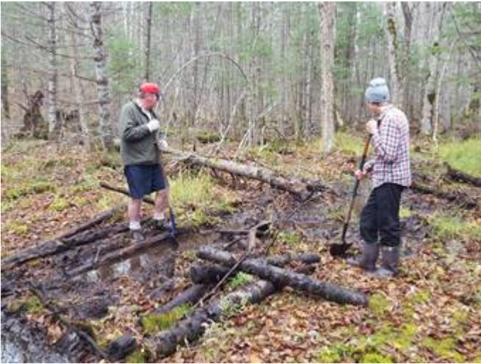
October: draining wet area on B loop, and applying corduroy
