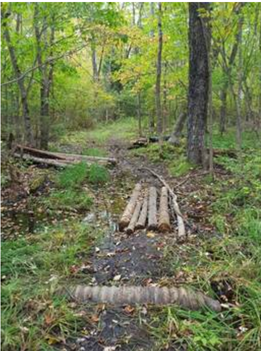
September: adding corduroy, culverts, and sand to C loop wet spot (before and after)
